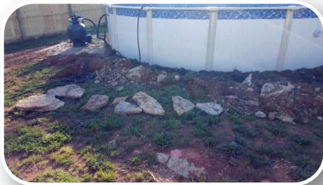
Some jobs have a little rock in the ground when we dig, so be aware that your yard could have the same. It is important for the bottom of the pool base around the outside to have dirt pushed up around it to help contain the sand.
